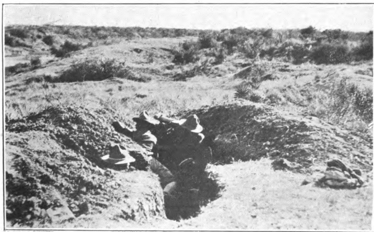
Trench for Lewis gun in process of construction
