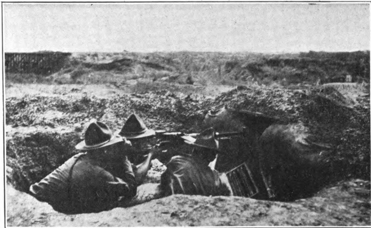
Light type machine gun emplacement. Only sufficient room is necessary for three men.
